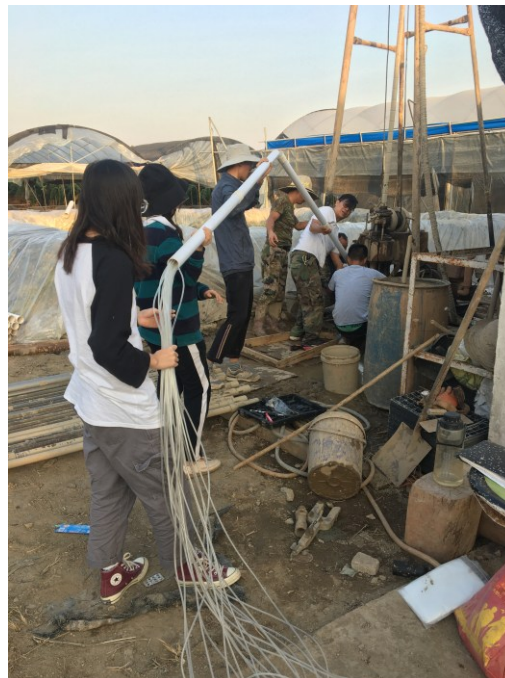
Figure 7 A 20-tube groundwater sampler system is installed in the Quaternary aquifer-aquitard system in the Pearl River Delta, China. The deepest tube reached the depth of 78 m.
