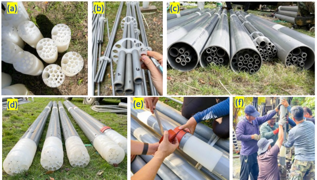
Figure 3 A HKU 18-depth dual purpose system was installed into interlayered sandstone and shale geological system in Chiao-Tung University in Taiwan to study slope stability. (a) Holes of ports are marked and numbered. (b) PVC tubes (piezometers) are numbered and organized using holders. (c) Organized PVC tubes are inserted in large protective pipes. (d) Ports are connected. (e) Seals are wrapped at desired depth. (f) The system is inserted in the borehole section by section.
