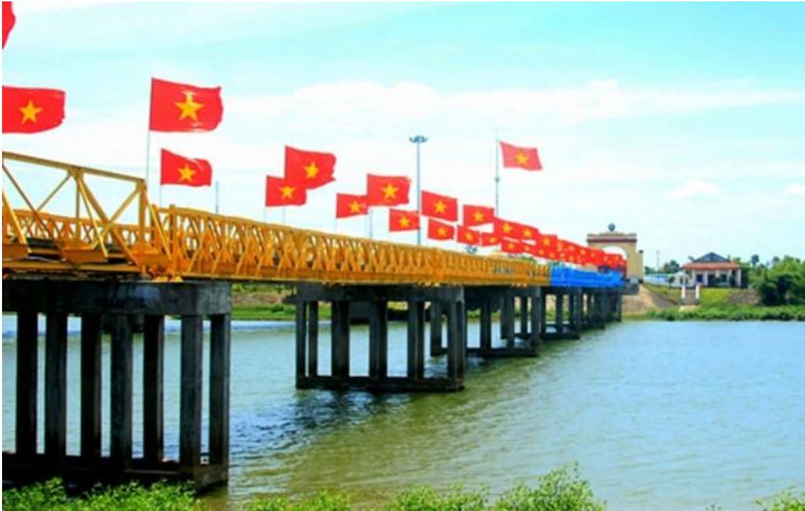
Figure 2.14 Hien Luong Bridge
